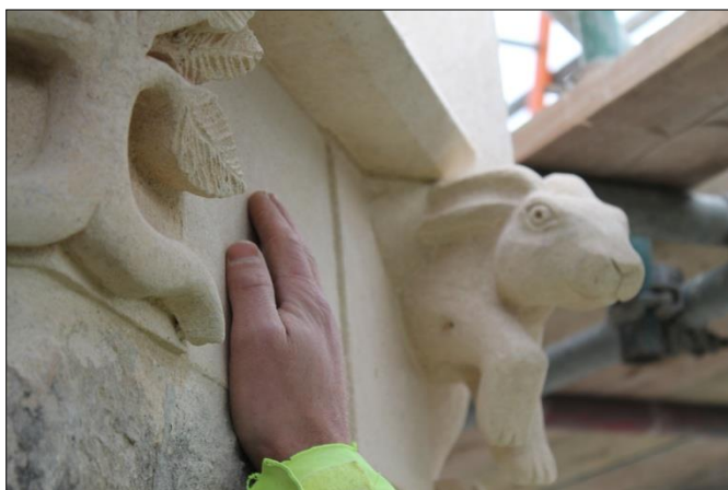
All in hand – the corbels in place.
