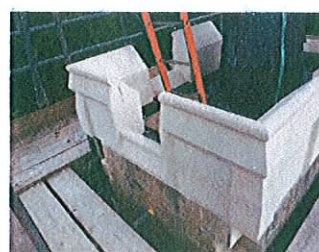
The completed tower parapet stones
