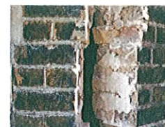
The quoin stones being cut out
