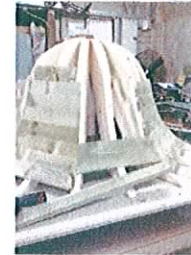
View showing new timberwork on turret
