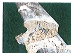
The copings were cut out
