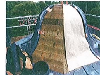
The new leadwork on the turret
