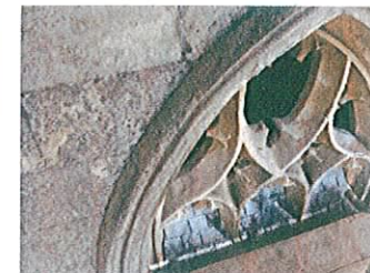
View of the south tower showing badly cracked tracery
