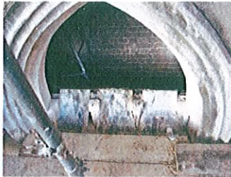
View of tracery being cut out
