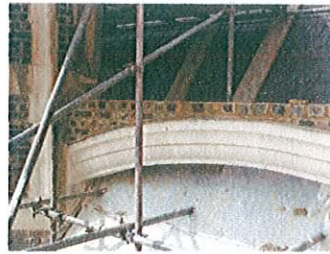
When the arches are completed the timber can be removed
