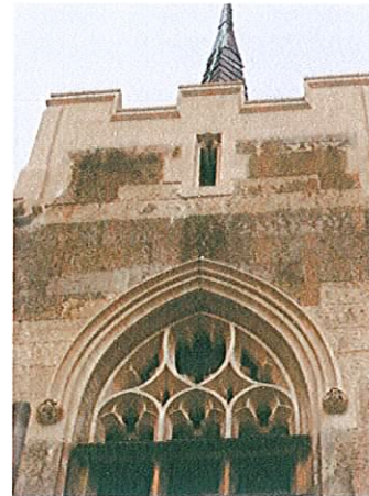
The completed tower parapet stones and tracery
