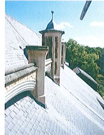
The completed south aisle arches
