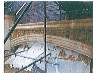
View showing the brick infill and completed copings
