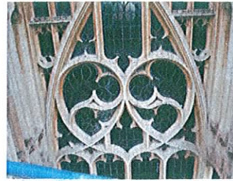
Typical views of the window showing the decayed leadwork to the tracery
