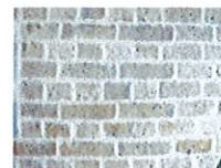
Newly pointed brickwork
