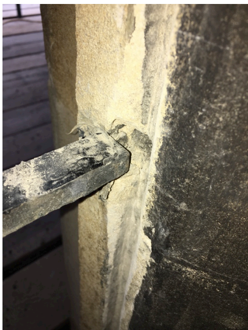
Figure 3 Typical views of ferementa showing that they are in perfect condition
