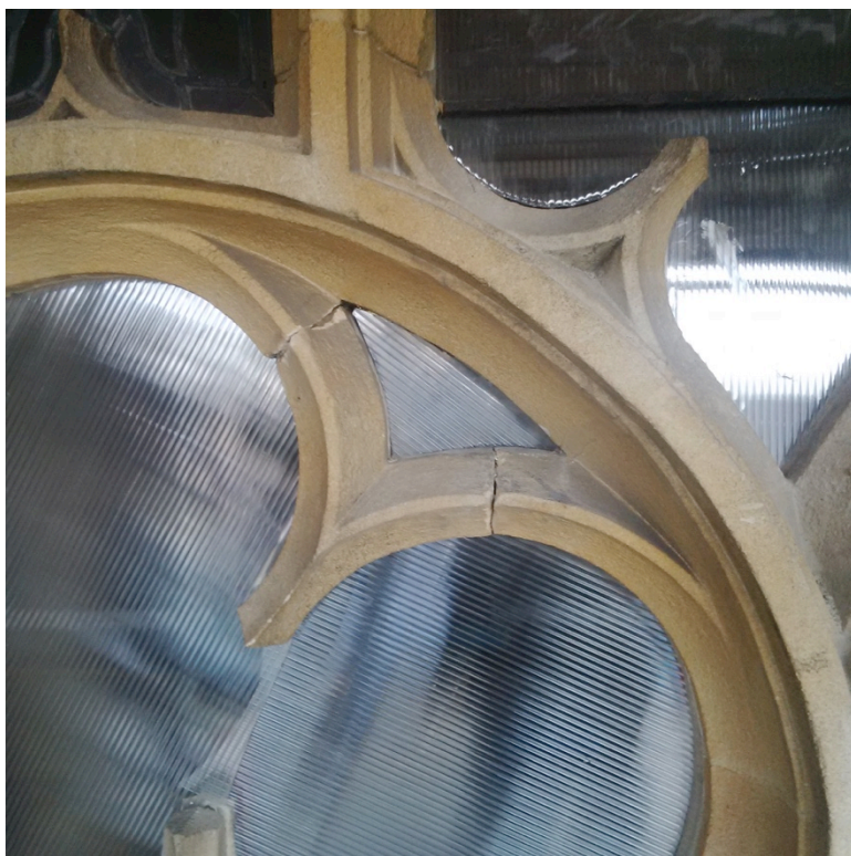
Figure 2 Typical view of tracery with temporary glazing
