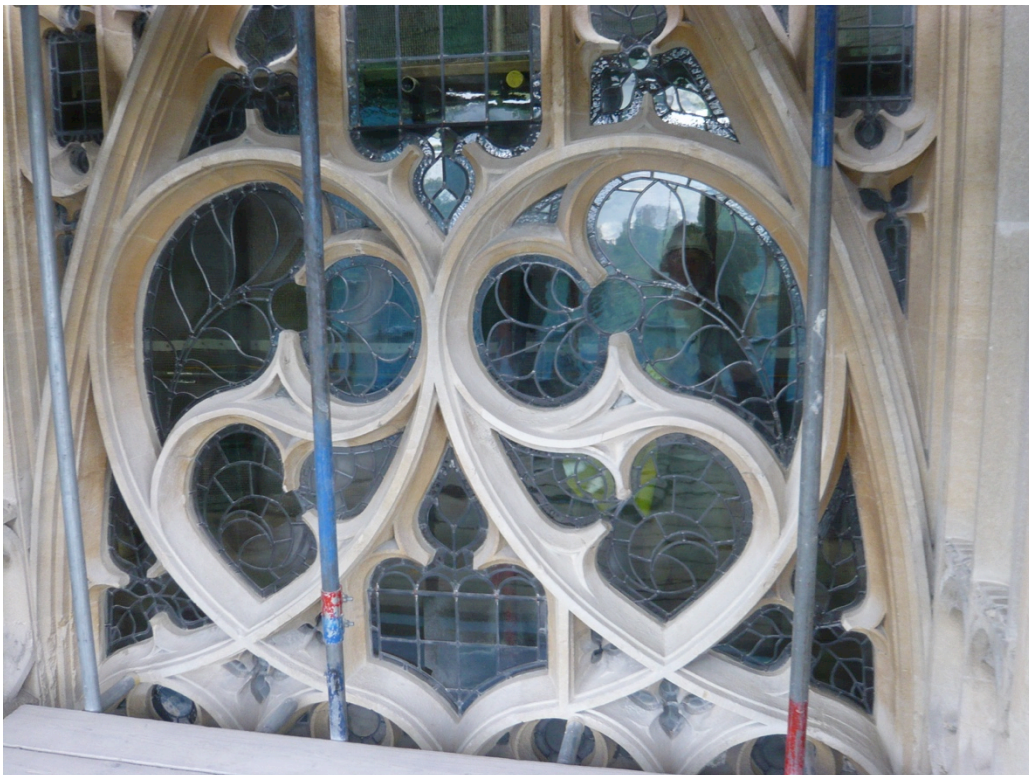
Figure 8 internal and external details of completed tracery glazing
