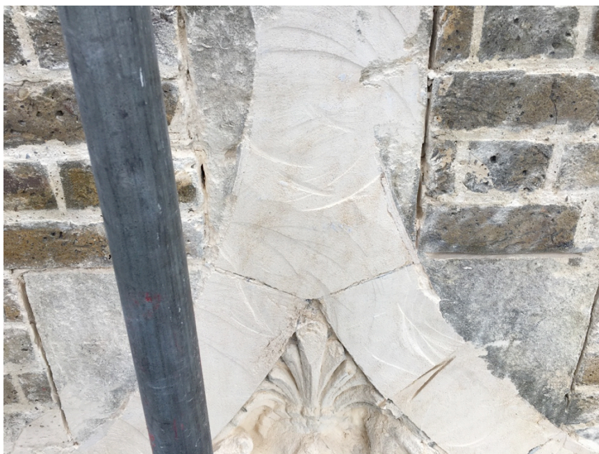
Figure 5 view showing apex of hood moulding cut out ready for replacement
