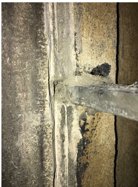
Figure 3 Typical views of ferementa showing that they are in perfect condition
